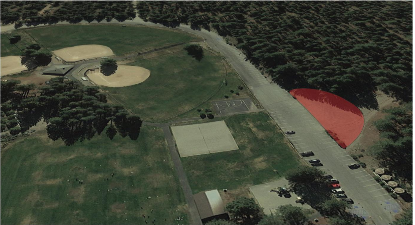
Proposed Parking Improvements to Prior Disturbed Area - Shady Rest Park - Winter Closure Area
